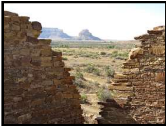
Breaking down walls
